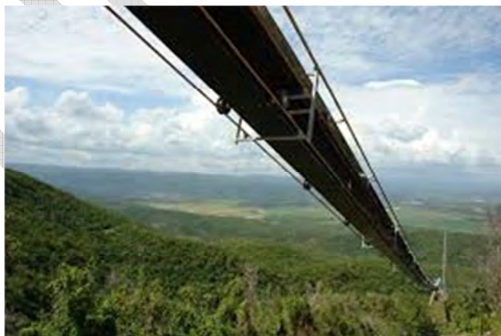
Figure 23 Typical Rope Conveyor System
