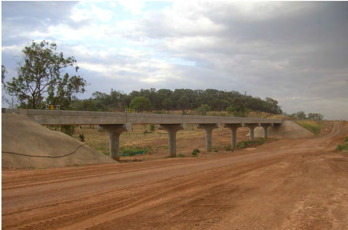
Figure 34 Typical Viaduct Using Prefabricated Components
